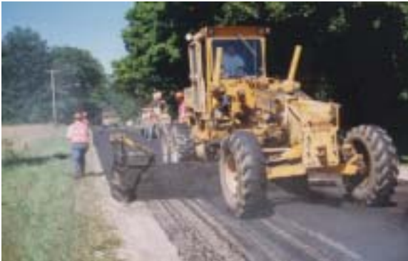
Figure 11. Grading foundry sand
