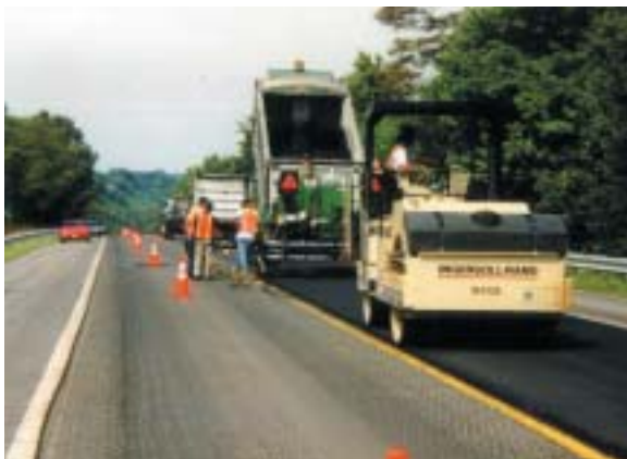
Figure 17. Construction of HMA pavement
